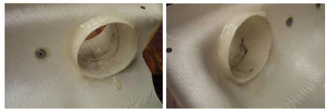
**Figure 37. Air Filter Box Plumbing – Incorrect** Correct plumbing – sharp lips & abrupt corners rounded & smoothed off.
