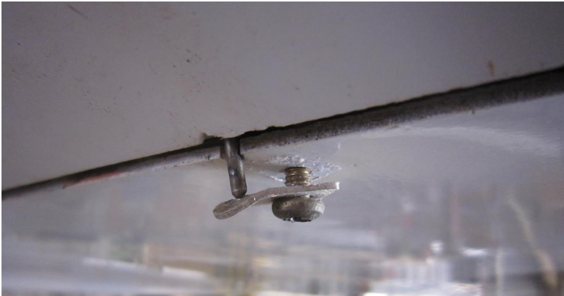
Figure 26 - Hinge pin unlocked
