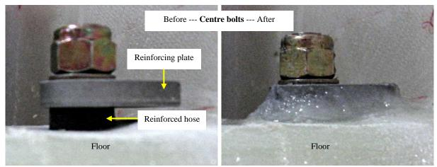
Tighten each nut until the first thread on the bolt is just visible above the top of the nut — at this point one side of the reinforcing plate will be very close to the cabin floor and the reinforced hose will be compressed to roughly half of its original thickness and will have formed to suit the shape of the floor so it will completely seal the bolt from any flock.
