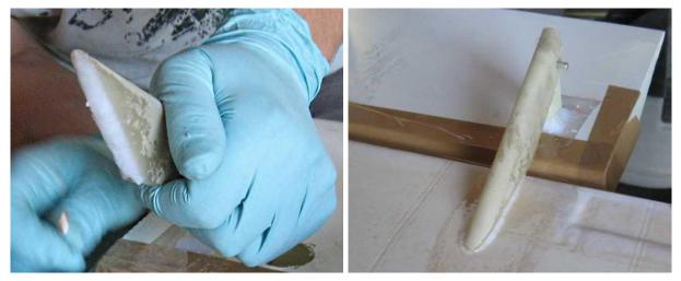
Place each bracket: holding the bracket clear of the wing, insert the bolt through the bracket and the bush, then let the bracket rotate down to the wing. Do this for each bracket.
