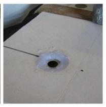
Clean away any dust then sand and test fit the quick drain body.
