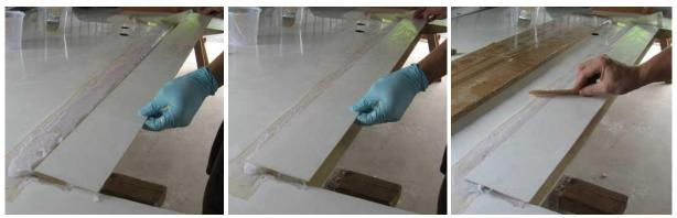
Fit the pre-mould strip into place – position carefully slightly above the final location and then press gently forwards and then down into place. Wipe away any excess flock.
