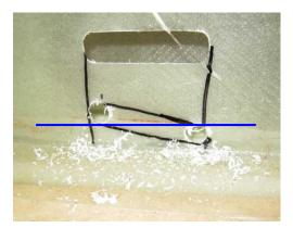
This slight upward angle allows a smooth cable run
