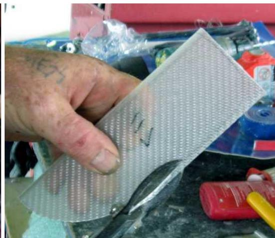
Next the front air dams will need to be cut to size. Take the length of glass fibre sheet with the curved edge, hold it against the rear of the duct inlet with the curve towards the top rear of the duct and mark around the bottom of the duct then cut to shape as shown above.
