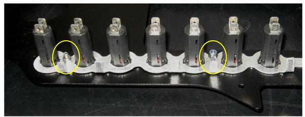
Drill through the 2 mounting holes in the earth busbar between the circuit breakers and bolt the busbar to the panel with 2 M4 screws and Nyloc nuts (shown circled above). Don't tighten the nut closest to the centre of the panel just yet (shown as the right hand nut above); the master earth will fit under this later during the wiring process.
